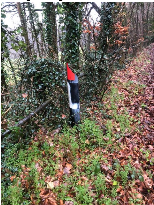
Damaged finger bollards on the Cothelstone Road
